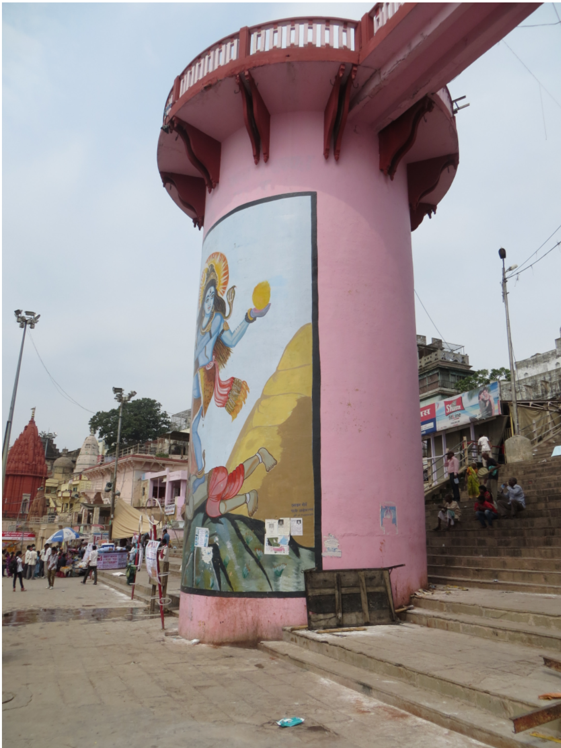
Rajendra Prasad ghat sewage pumping station (one of five ghat pumping stations that send sewage running underground toward the river back to the main trunk line and on to Konia pumping station)
