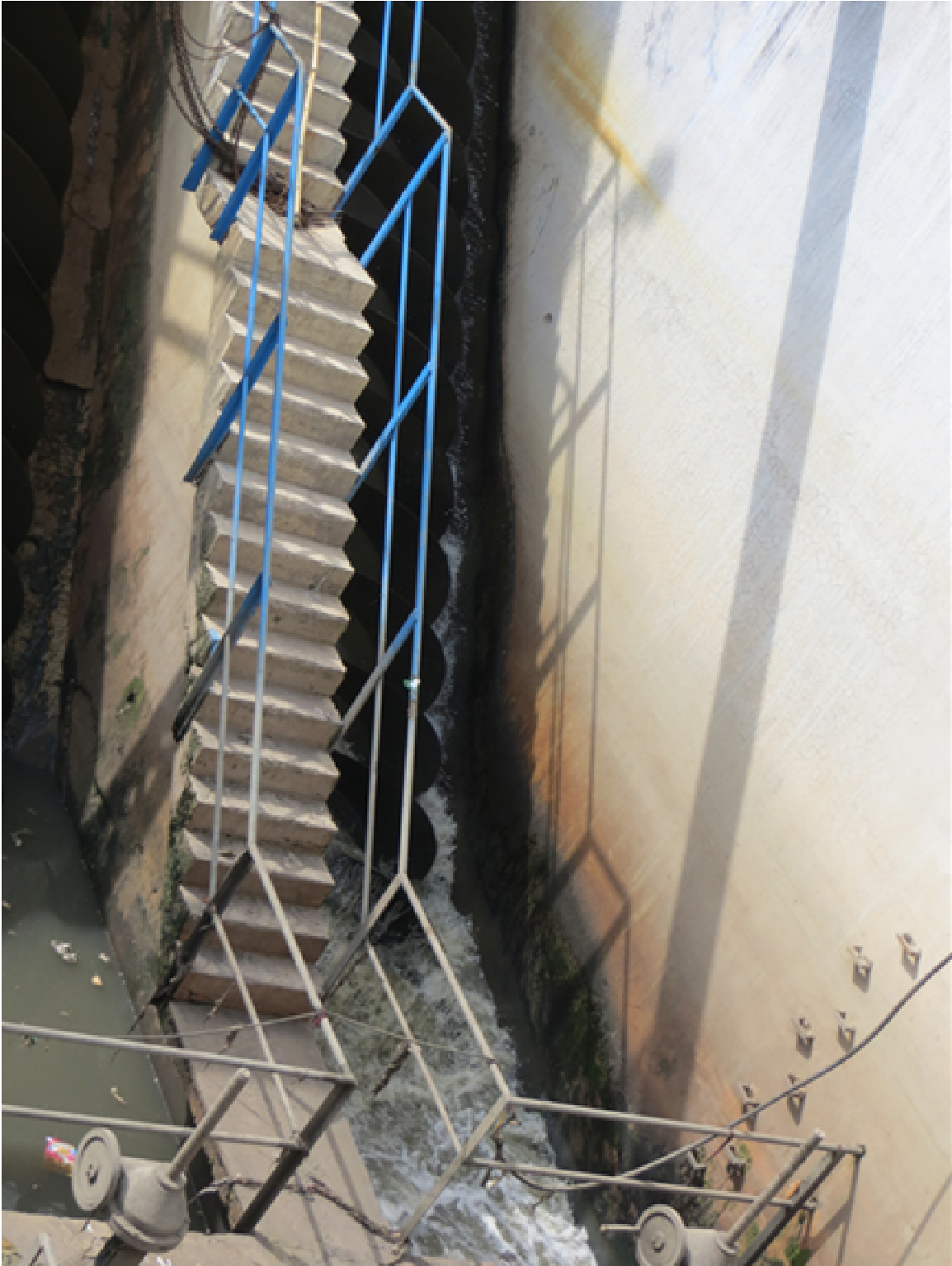
Another shot of Konia sewage pumping station with only one screw pump working.
