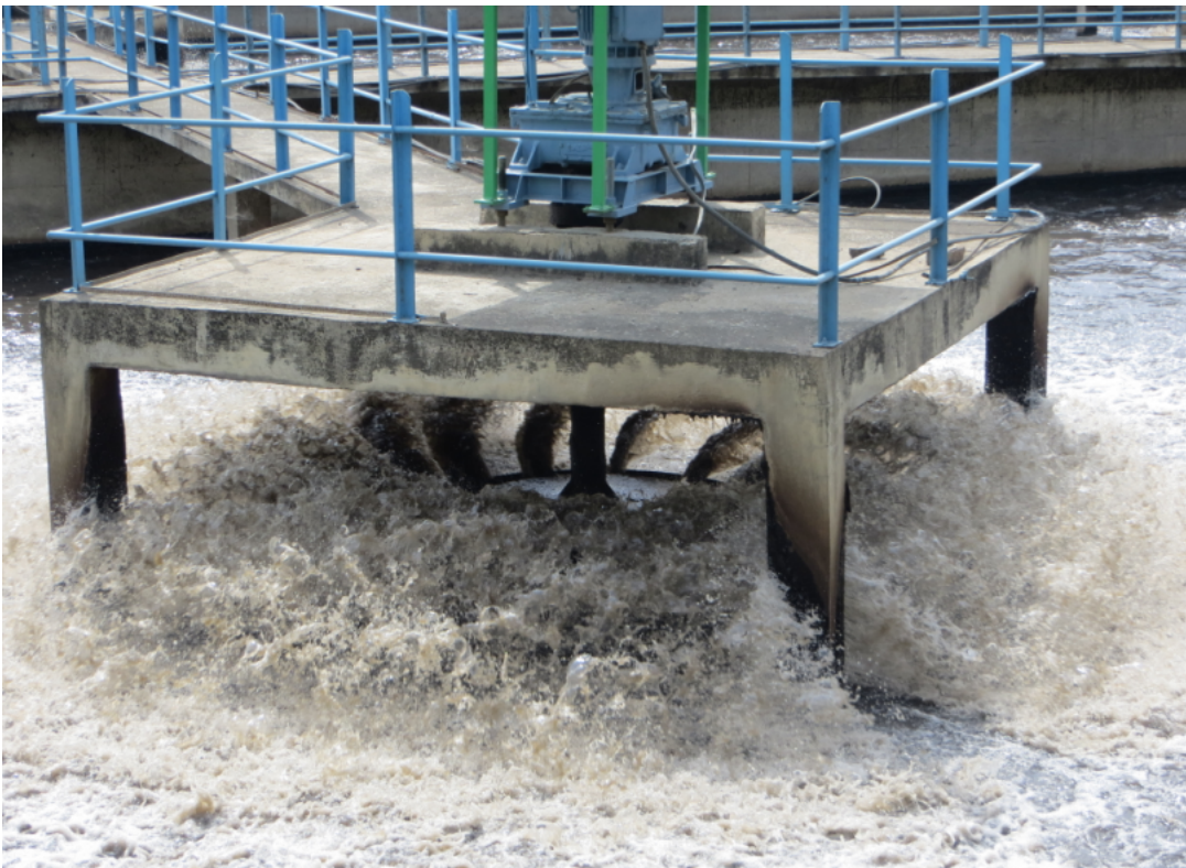
Low efficiency splash aerators in the aeration basin
