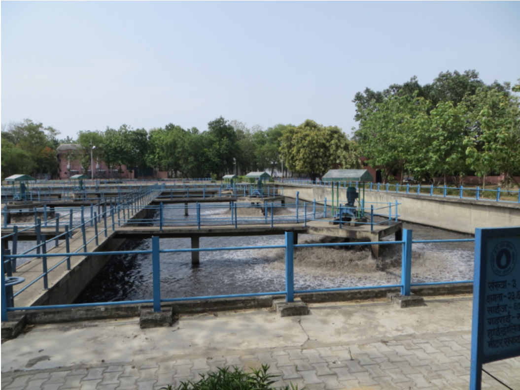
Aeration basins at the Dinapur sewage treatment plant.
