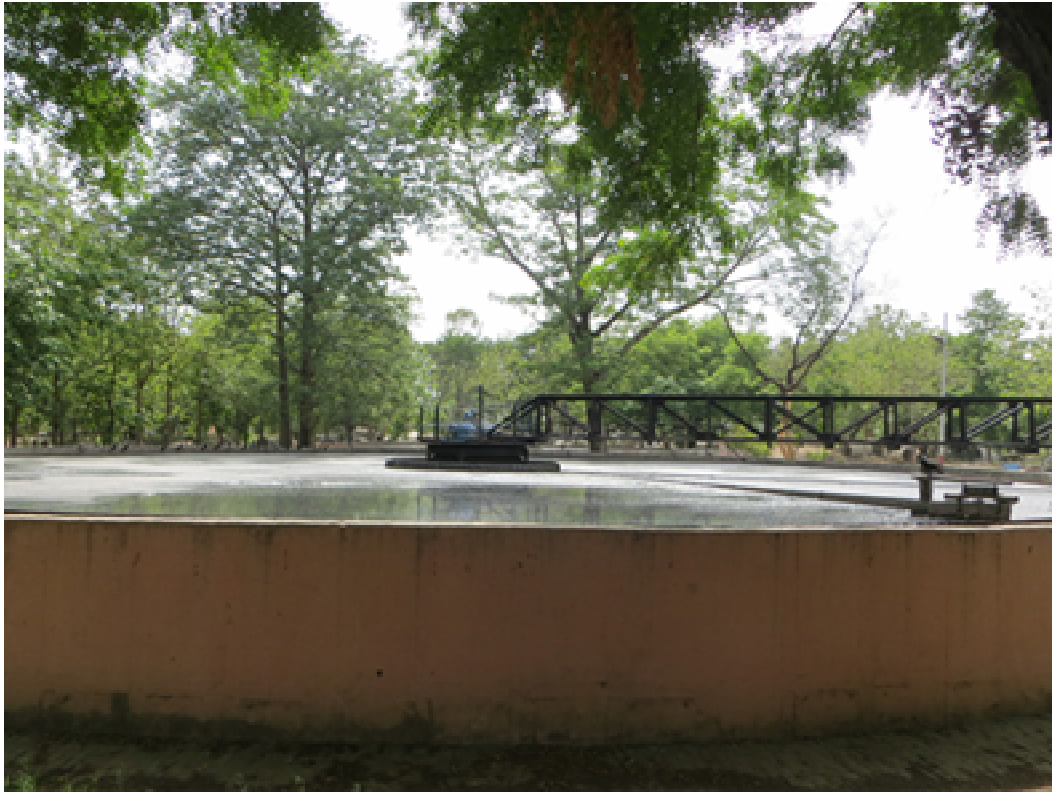
Secondary clarifier at the 80 MLD Dinapur sewage treatment plant.
