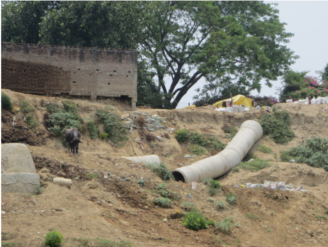
Sewage pipeline damaged by the flood of June 2013 but not repaired. When it was built, it was the pipeline to nowhere. There was no treatment plant constructed at its terminus in Ramana Village along the river bank and upstream of the Nagwa drain.
