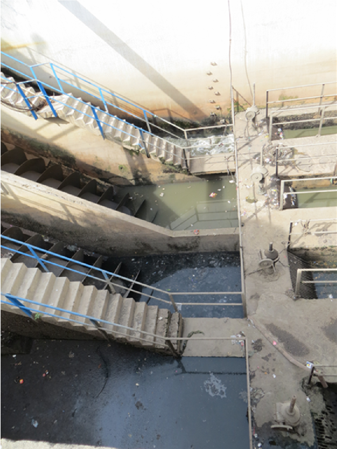
Konia sewage pumping station. Only one screw pump is working.
