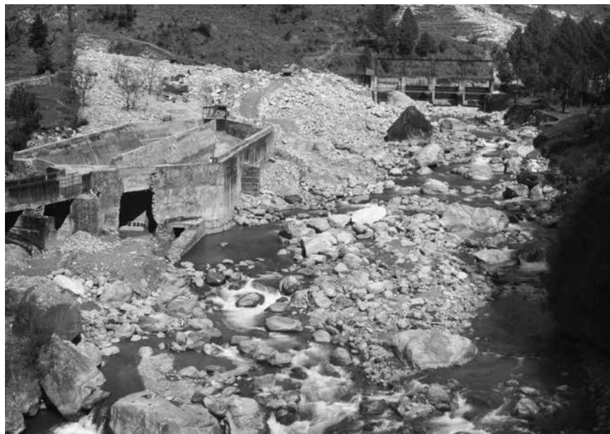
The damaged Jakhni-Vanala HEP damaged by bed-load movement
