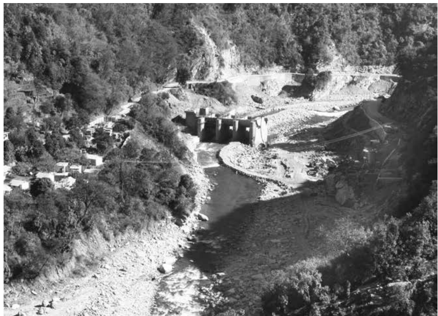
The Singoli-Bhatwari HEP that is now stranded at one side of the riverbed
