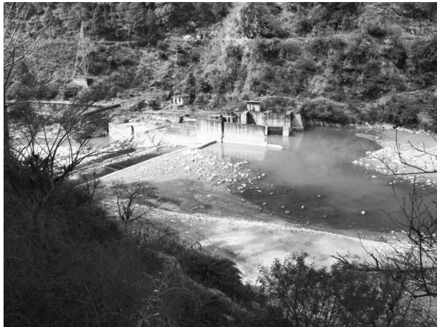
The small Rajwakti reservoir completely silted over
