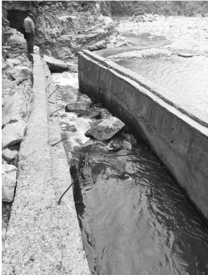
The broken and blocked fish ladder at the Larji dam
