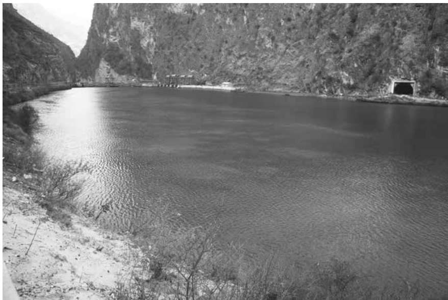
The Larji dam reservoir filled with sediment. The sediment shoals are clearly visible
