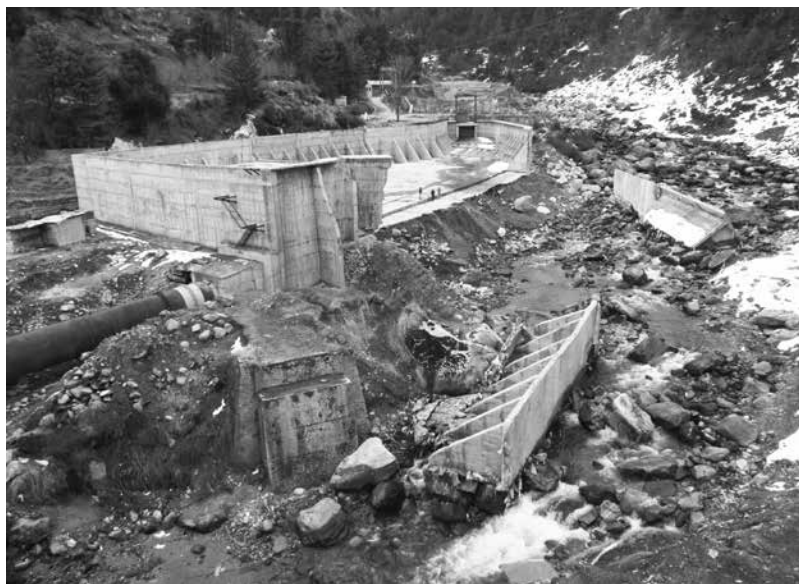
The collapsed Alleo sedimentation tank
