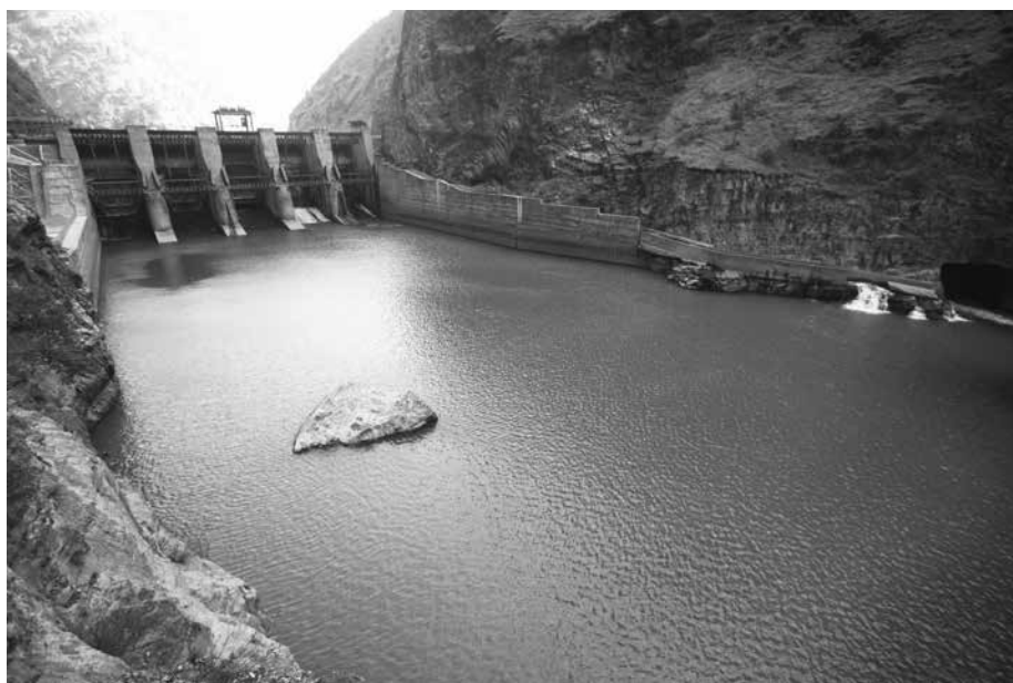
Downstream of the Larji dam. Broken-down fish ladder visible on the right bank in the photo
