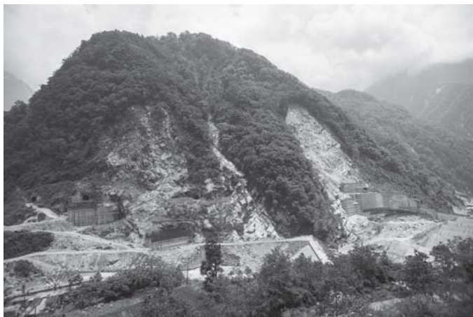
Photo from SC-NBWL committee report has this caption: Construction of the Teesta III project at Chungthang on the edge of Khangchendzonga National Park proceeding without SC-NBWL clearances. Note the extensive forest cover and large landslides at the site.
