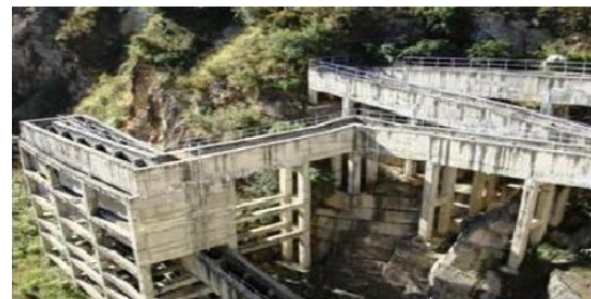
Fish Ladder on 60 MW Kurichhu Dam in Bhutan for migration of Golden Mahseer built by Indian NHPC Photo: drukgreen.bt
