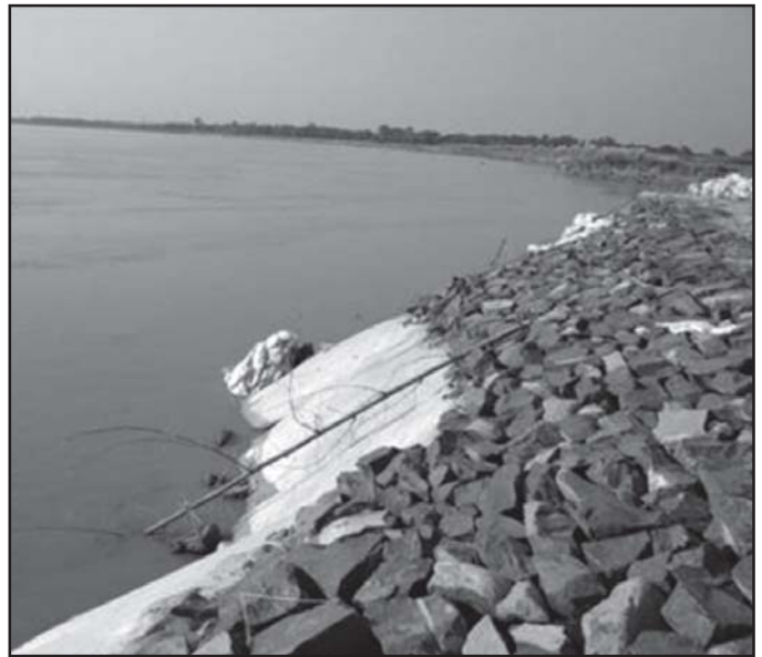
Washing away erosion control measures at Chow Bahadurpur downstream FBP Photo: Author
