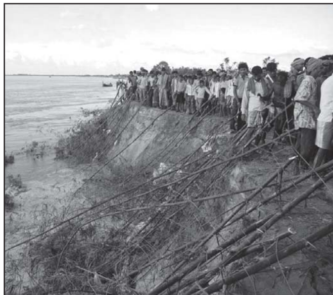
Bank Erosion and Embankment breach at Hiranandpur Photo with thanks: Soumya Desarkar
