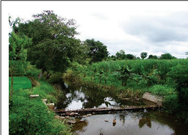
Figure 7: check dam and loss of riparian vegetation. Site: Beegar, Yellapura
