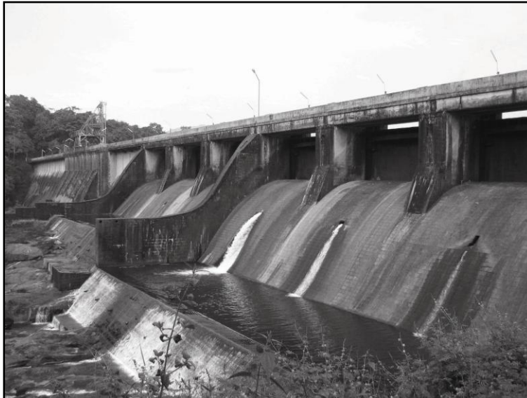
Peringal Dam: Photo source: CPSS
