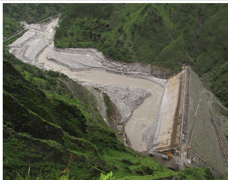
Figure 1 The Dhauliganga Hydro-power dam, after being flushed of bed-load sediment
